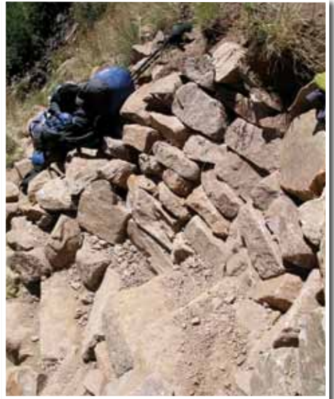
Chicago Basin rock staircase and retaining wall
