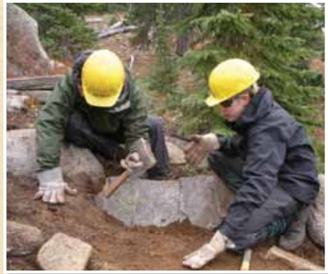
High Mountain Institute summer campers build erosion control features on Mount Yale
