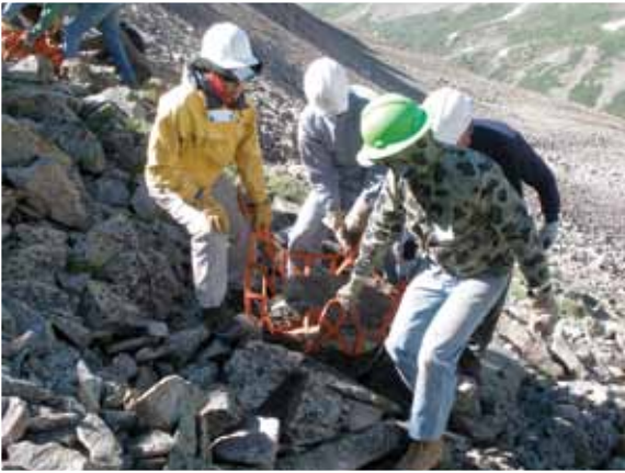
Moving rocks for use in trail structures
