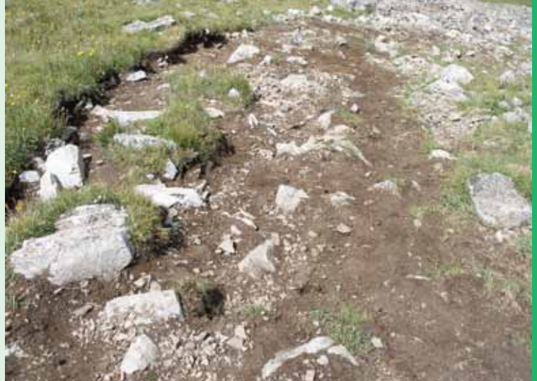
Volunteers for Outdoor Colorado crew stabilizing and restoring this eroded area with vegetation plug transplants
