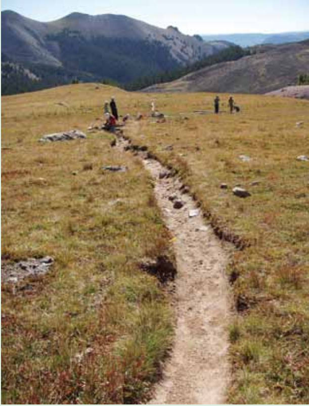
Colorado College students install waterbars and fill soil to restore natural contours and minimize trail erosion at Uncompahgre Peak
