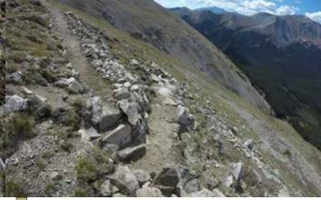
Rock walls and staircases help stabilize the tread on a steep portion of the new trail.
