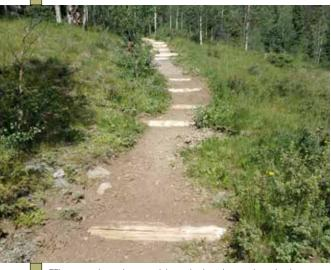
CFI increasingly uses logs to stabilize trails where there are limited rocks of sufficient size.
