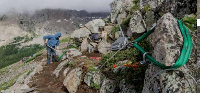
$Wade\ Frisbee\ uses\ a\ griphoist\ to\ carefully\ position\ a\ large\ rock\ into\ place.\ Photo\ by\ Eli\ Allan,\ www.eliswindow.net.$
