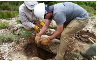
Placing a rock step on a VOC project on Redcloud Peak.
