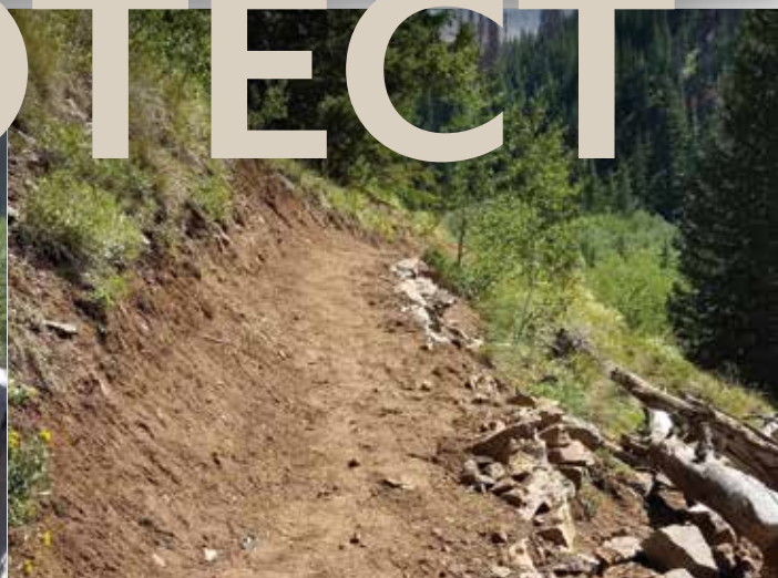
BEFORE, DURING, AFTER: A Volunteers for Outdoor Colorado team stabilizes the critical edge of the Redcloud/Sunshine trail, which is particularly subject to collapse due to the steep cross slope.
