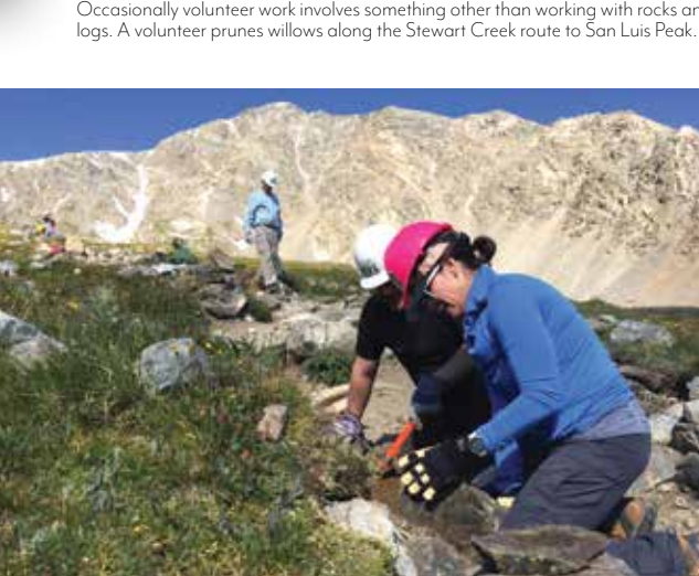
Volunteer Priscilla Clayton helps position a rock in a retaining wall along the popular Grays and Torreys route.
