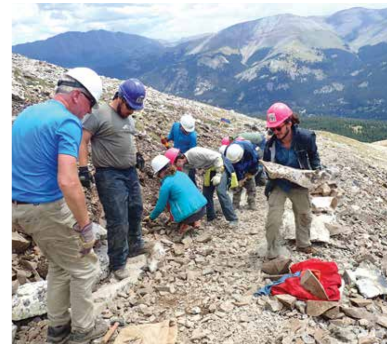
Volunteers haul rocks to build a backwall to control erosion.
