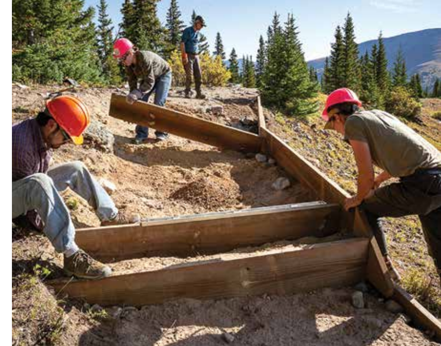
Volunteers on the NFF-sponsored project install a dimensional timber structure. Photo by Cameron Miller Photography.
