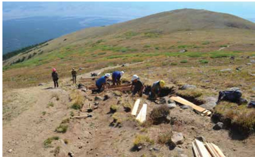
WRV volunteers install cedar planks to control erosion on the Elbert "cat's claw."
