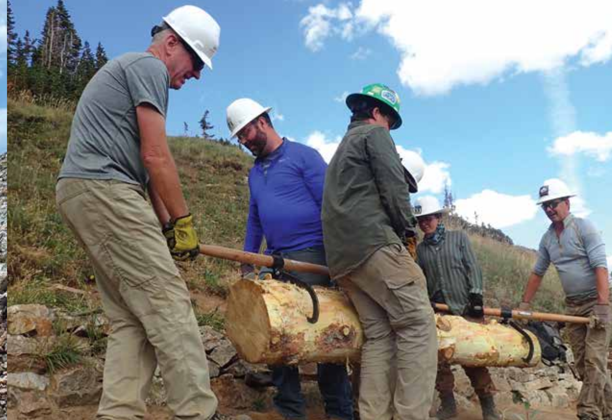
Six people move a large log into place to stabilize the critical edge of the trail.
