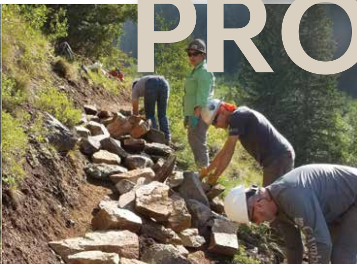
BEFORE, DURING, AFTER: A Volunteers for Outdoor Colorado team stabilizes the critical edge of the Redcloud/Sunshine trail, which is particularly subject to collapse due to the steep cross slope.
