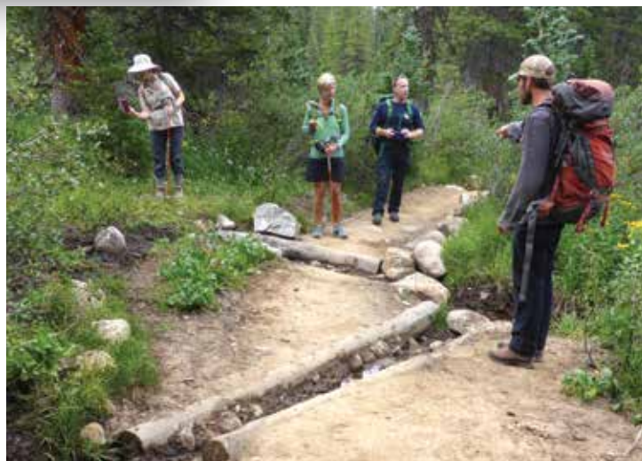
Project manager Eli Allan explains a drainage system installed to improve a muddy section of the approach trail to Columbia.
