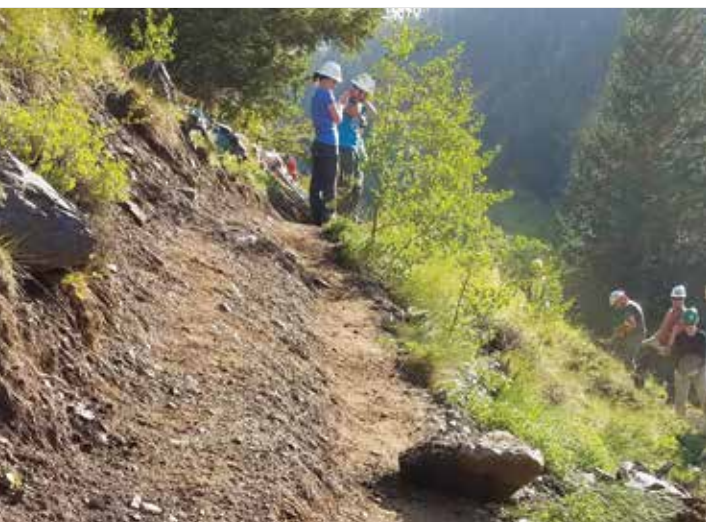
BEFORE, DURING, AFTER: A Volunteers for Outdoor Colorado team stabilizes the critical edge of the Redcloud/Sunshine trail, which is particularly subject to collapse due to the steep cross slope.
