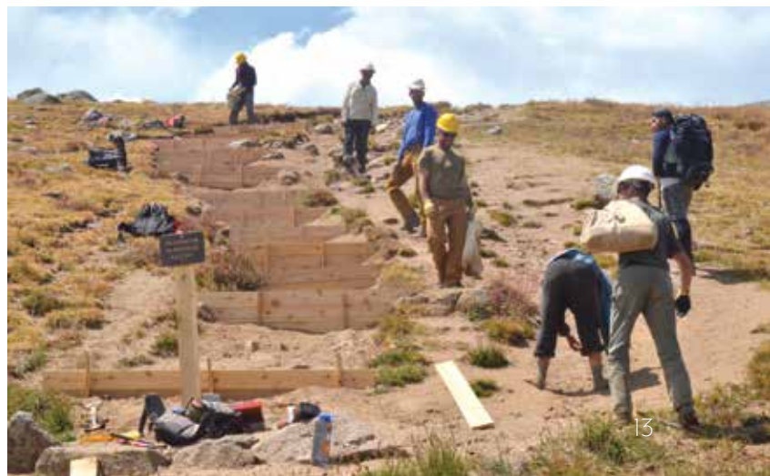
Volunteers haul soil to backfill the cedar plank retention walls to fill up the deep erosion scars.
