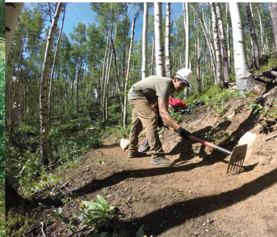
Addie Moncayo uses a McLeod to fine tune the lower Elbert reroute.
