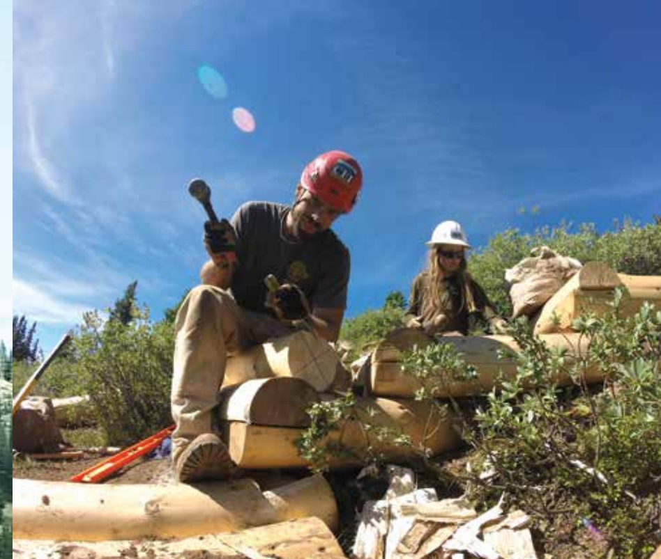
Justin Towers chisels out logs to be used in log staircases on Elbert.
