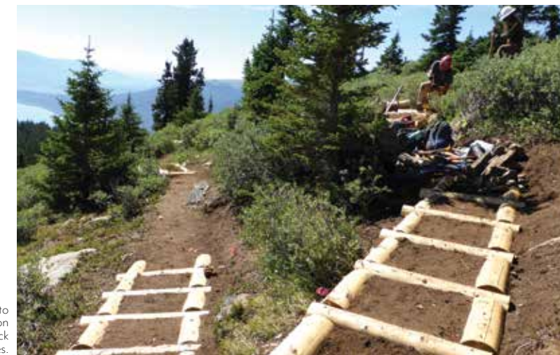
Addie Moncayo uses a McLeod to fine tune the lower Elbert reroute.
