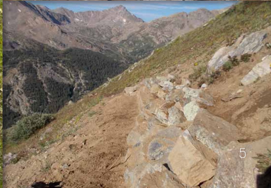
A volunteer from the Jaywalker program helps build a retaining wall on the North Maroon Peak approach trail as it climbs steeply out of Minnehaha Creek.
