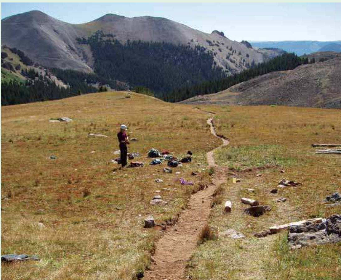
Colorado College students install waterbars and fill soil to restore natural contours and minimize trail erosion at Uncompahgre Peak
