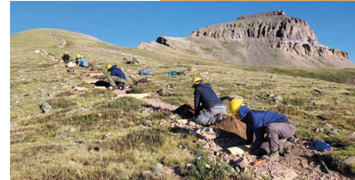
Members of the SCC youth corps crew install timber checks on the shoulder of Uncompahgre.
