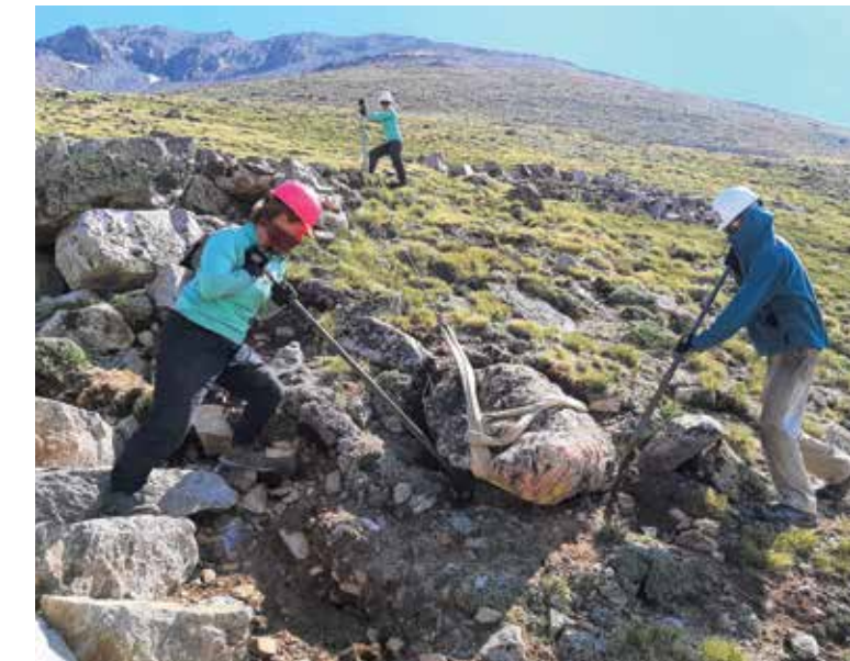
Crew members use a griphoist to carefully lower a rock into place in a multi-step staircase.
