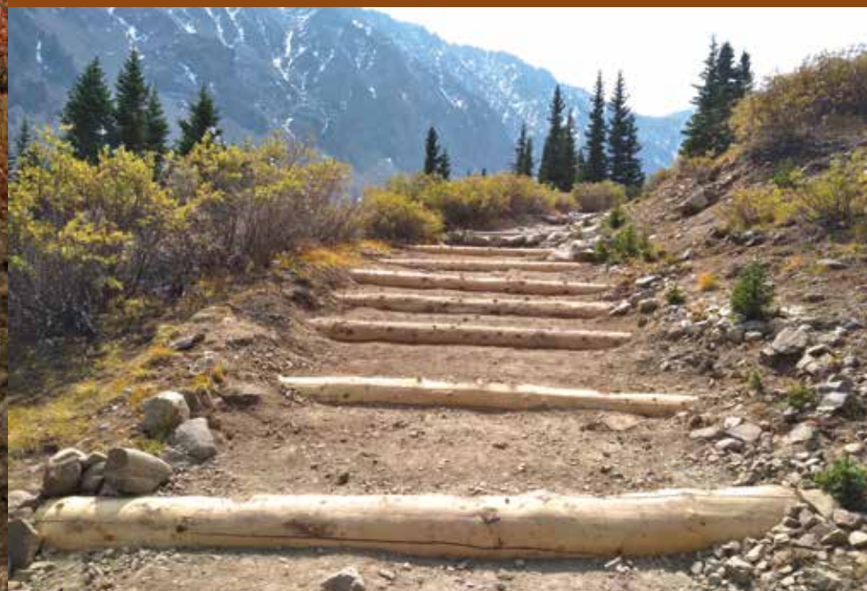
Some of the eight timber check steps installed.
