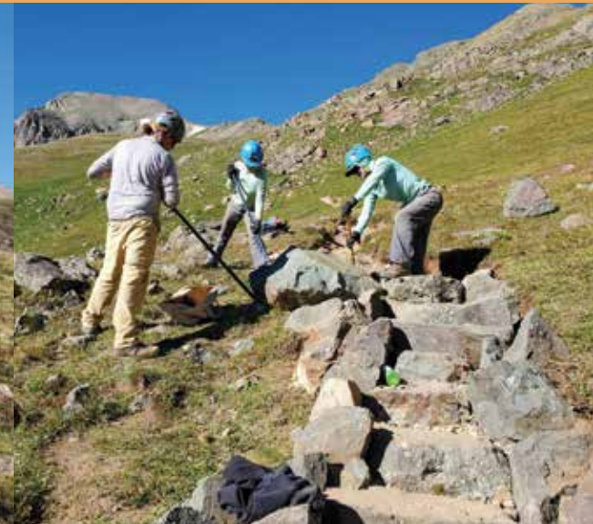
The Adopt crew installs a rock staircase high in Grizzly Gulch.
