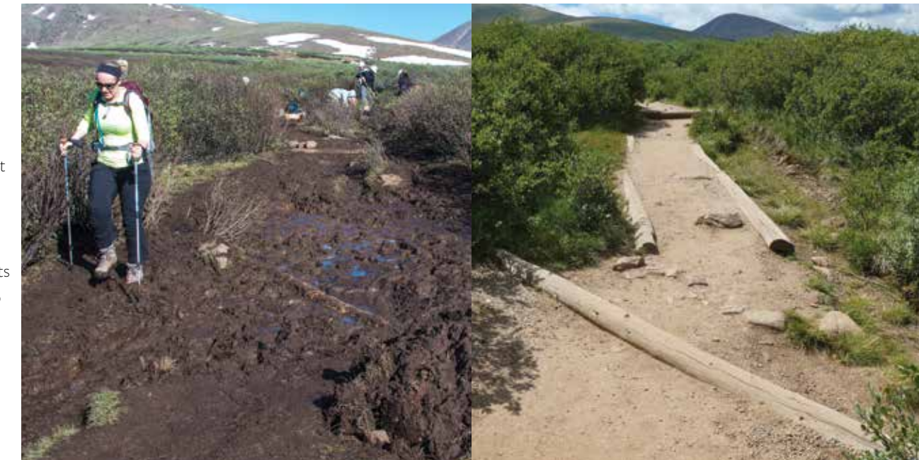
Over six years, willows have regrown and the elevated causeway is reducing impacts on the flat, wet, opening mile of the Mount Bierstadt summit trail.
