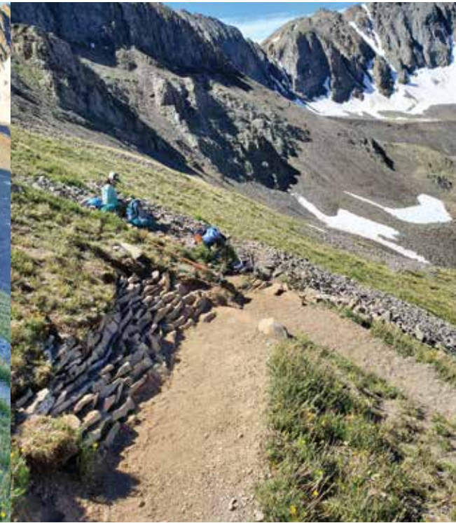
Before/After. A switchback in American Basin is fortified with a rock step and backwall.
