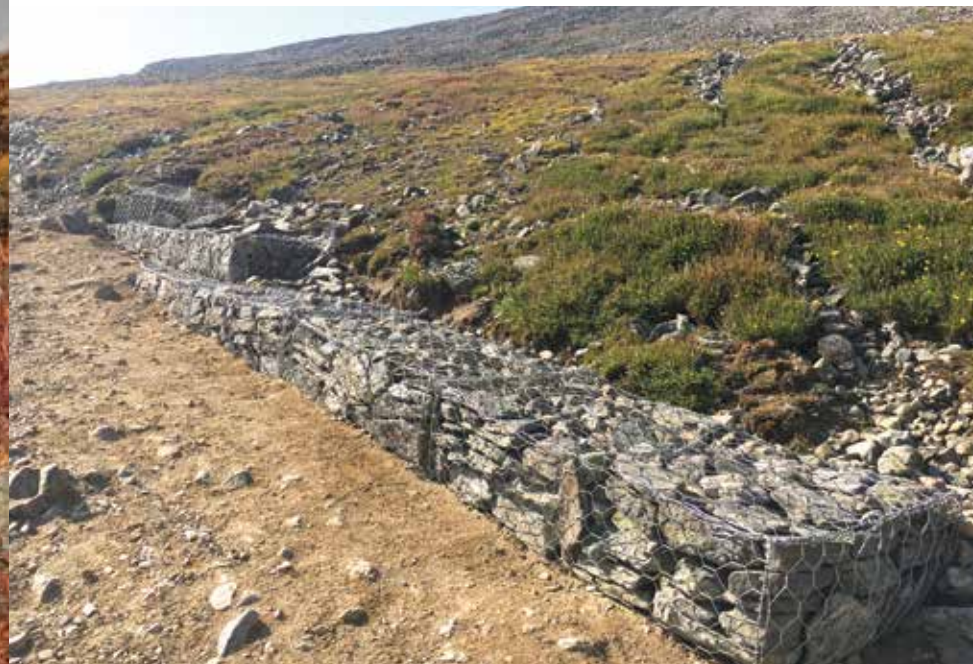
The completed section of gabion backwall protecting the tundra slope.
