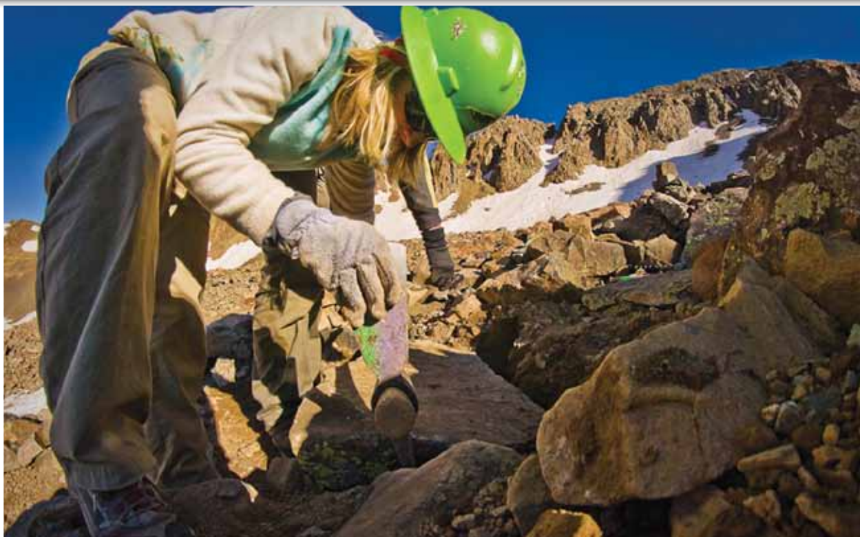
Roving Backcountry Crew member Danica Ivanovich places a rock step on the Mount Sneffels summit trail. Photo by Eli Allan, www.eliswindow.net .
