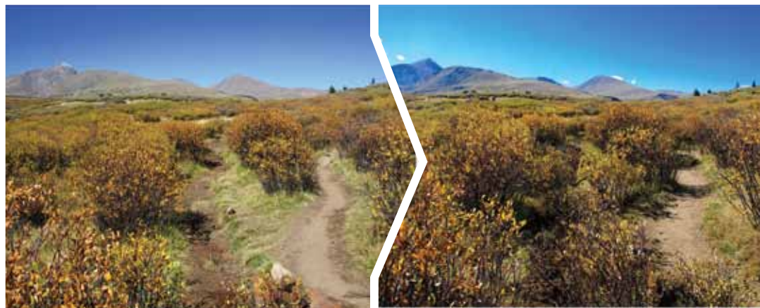
» Transplanted willows, grasses and rocks close off the left-hand braid following a service project.
